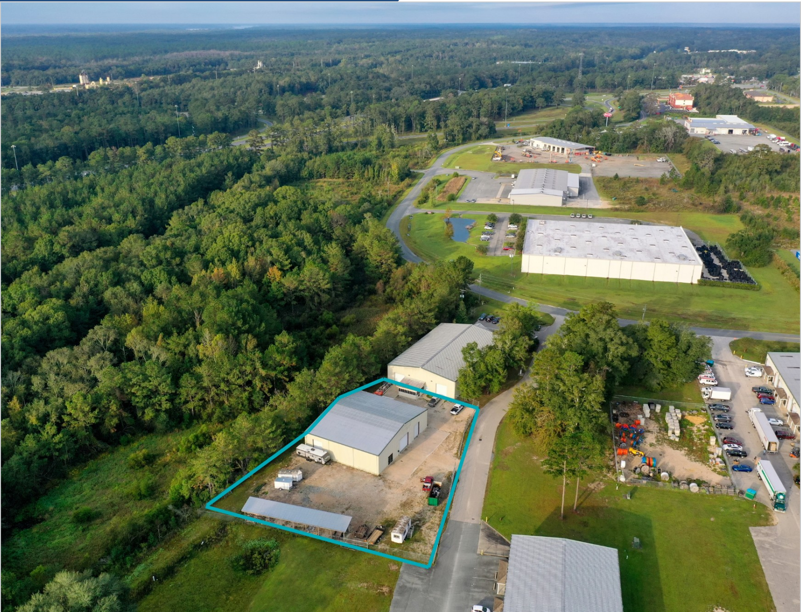
SUBJECT SITE OUTLINED WITHIN THE RAM BOULEVARD INDUSTRIAL PARK
