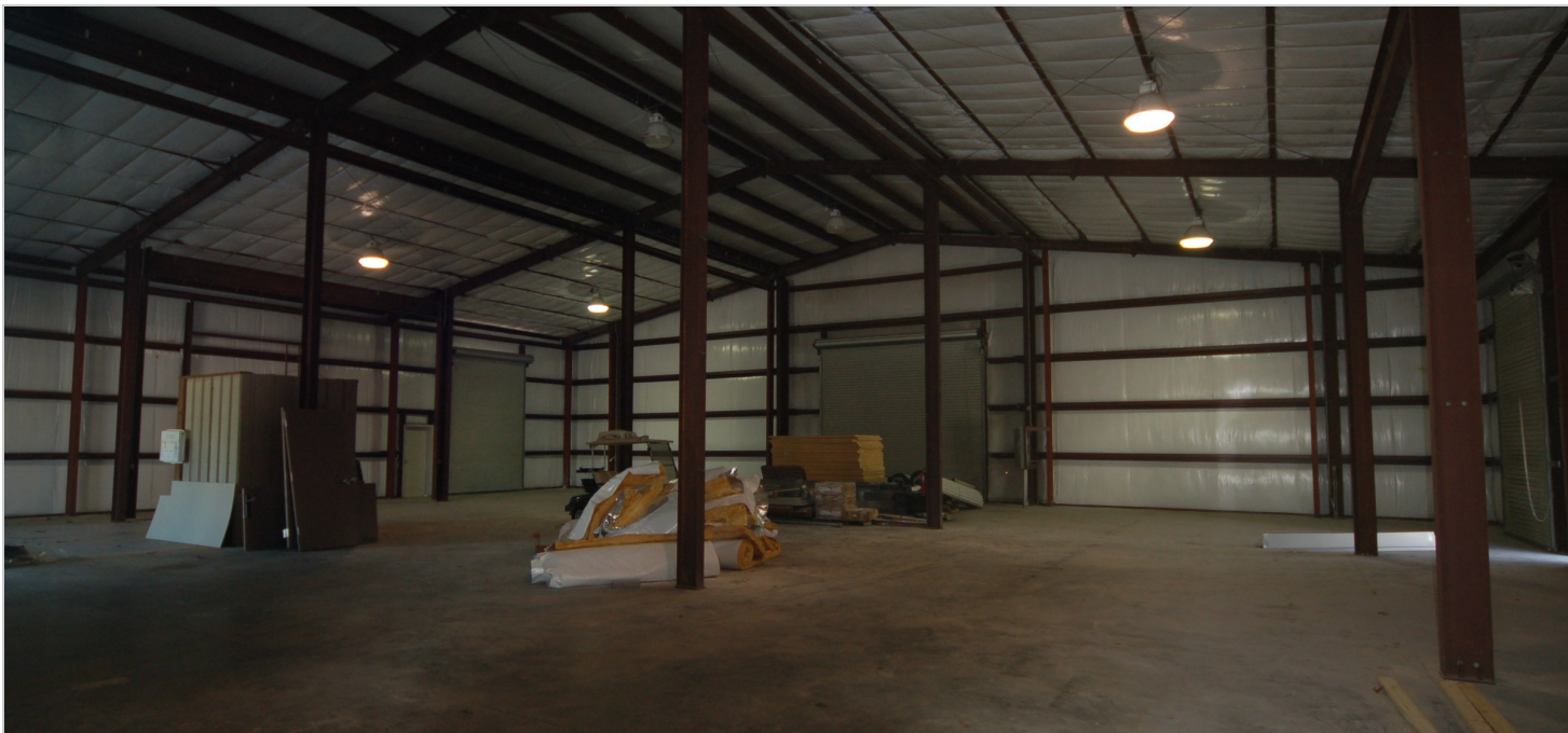
OPEN WAREHOUSE, CLEAR SPAN FRAMING AND 20 FT CLEAR HEIGHT
