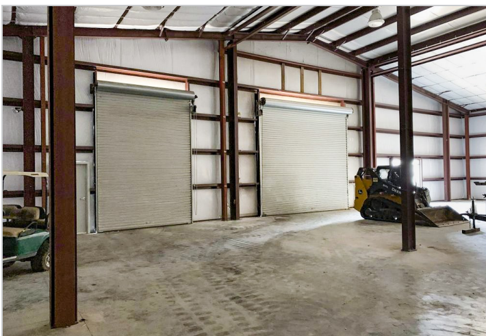
GRADE LEVEL DOORS FROM INSIDE
