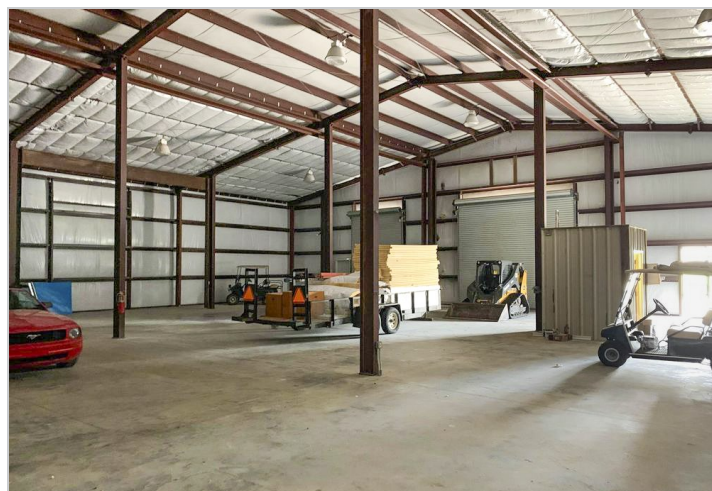
WAREHOUSE LOOKING ACROSS THE COLUMN LINE
