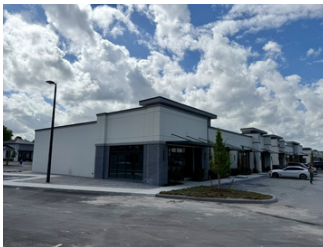
Corner elevation and surface parking field
