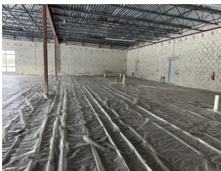
Grey shell interior – open-web steel joists and metal roof deck
