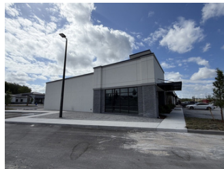
End-cap building form and brick base
