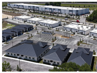
Lake Carter Exchange – aerial of the development
