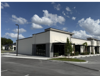
Storefront glazing along the frontage
