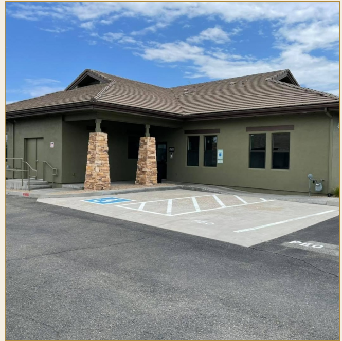
Building at 3623 Crossing Dr, Prescott
