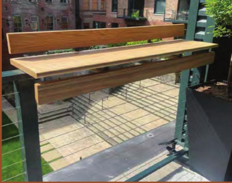
drink rail on railing at terrace deck
