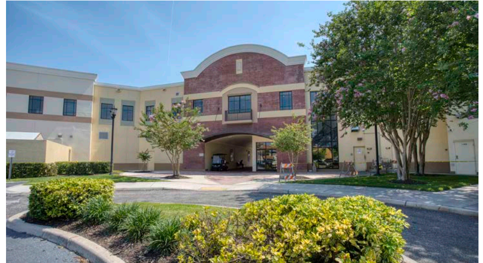
BUILDING N PARKING ACCESS
