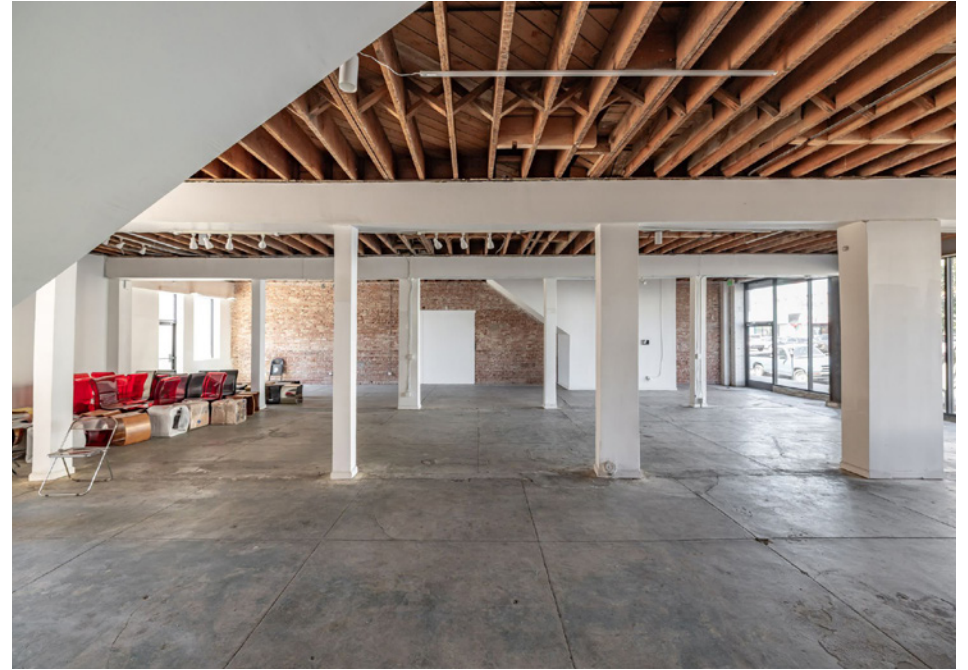
● Ground floor looking north toward N Western Ave
