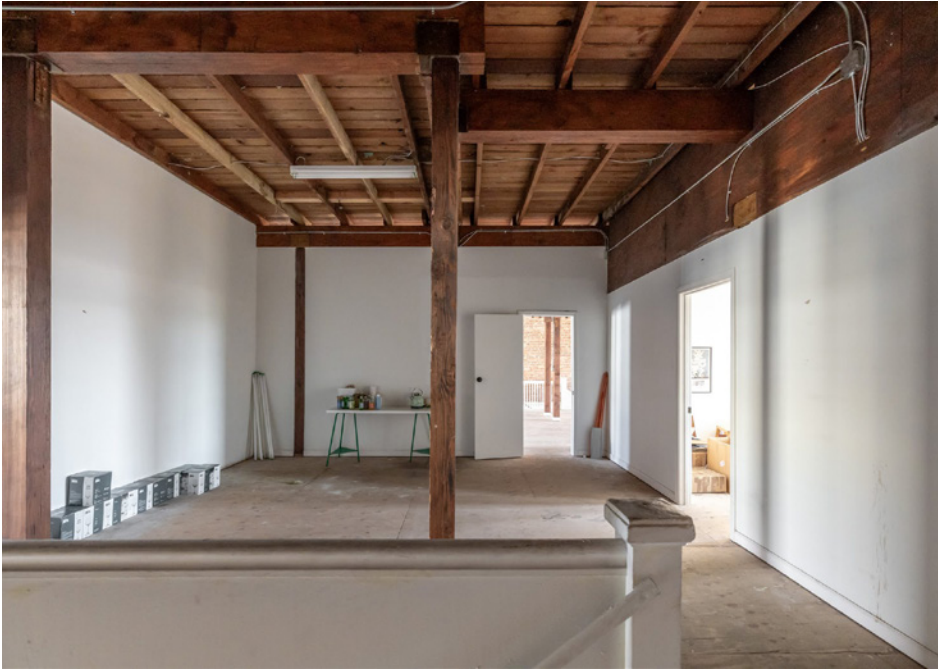
● Second-floor landing overlooking the temporarily demised office areas
