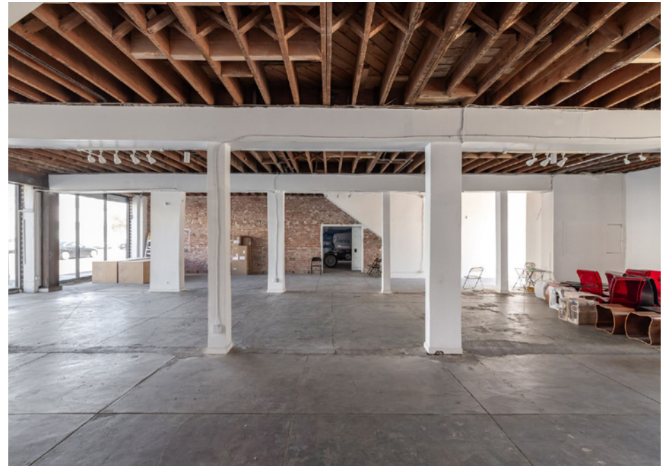
● Ground floor looking south toward the shared paseo with 619 N Western Ave
