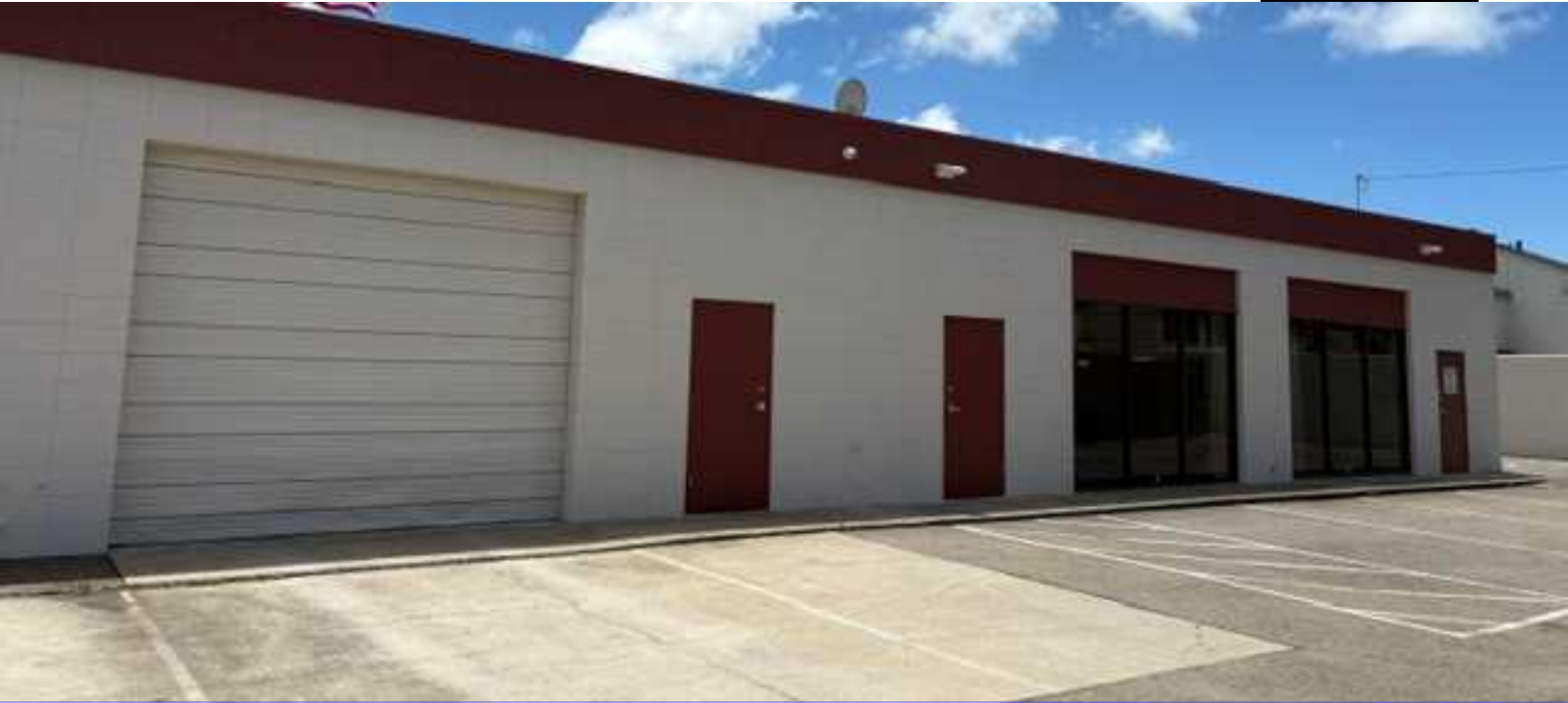
Rear of Retail/Service/Automotive Unit
