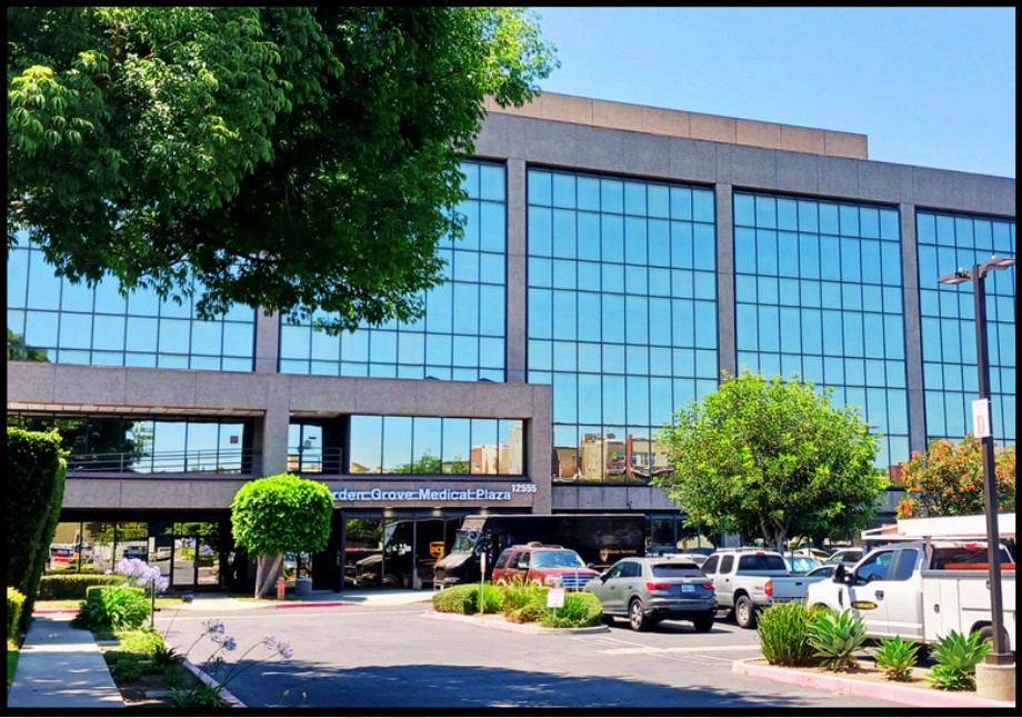
Parking Lot Entrance
