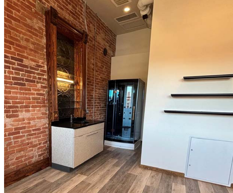
Water access and sink in Suite 216
