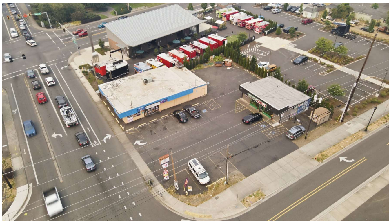
Aerial perspective showing the subject property within a high-visibility neighborhood retail setting.
