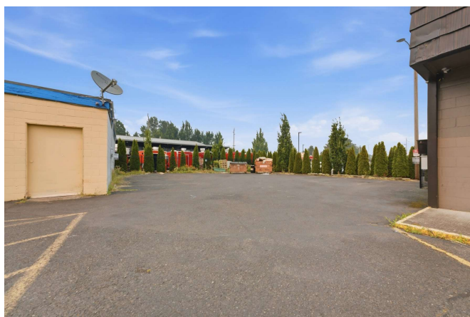
Rear/side parking and service area between the subject and adjacent property.
