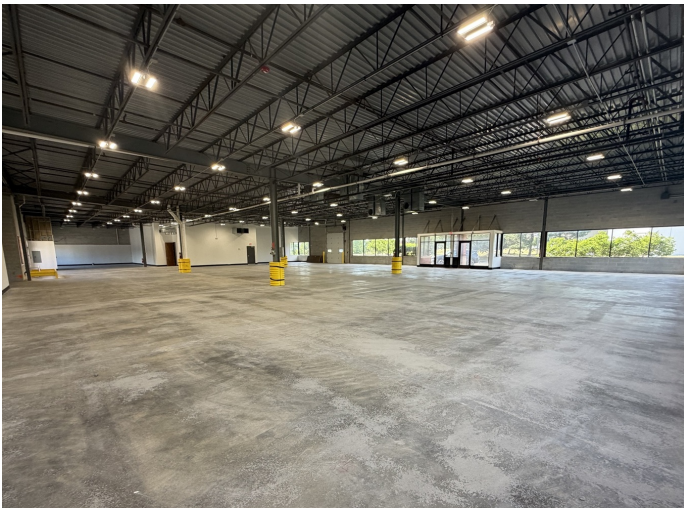
GRADE-LEVEL DRIVE-IN ACCESS
