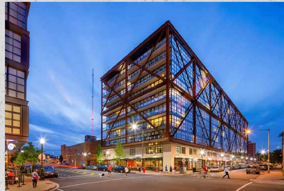
Atlantic Plumbing, Washington, DC
