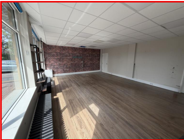
Picture shows ground floor office/retail area
