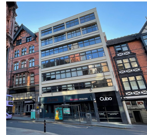
CUBO NOTTINGHAM Fenchurch House 12 King Street Nottingham NG1 2AS
