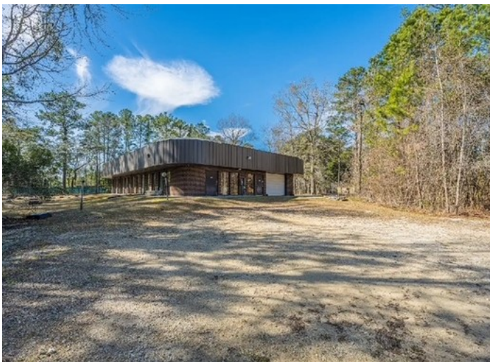
Rear building access and parking area
