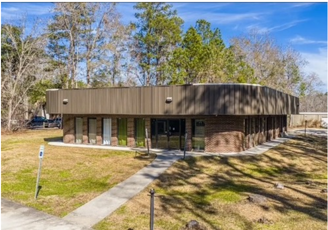
Front elevation and customer entrance
