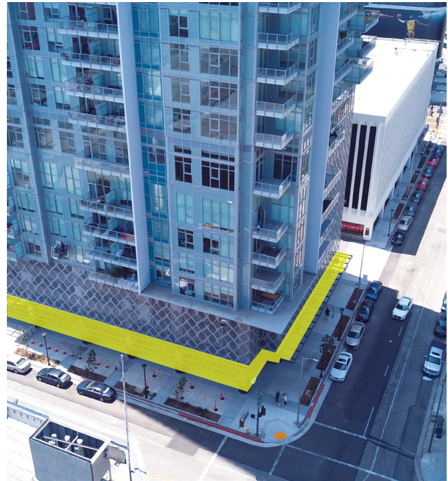
■ Building C Retail
