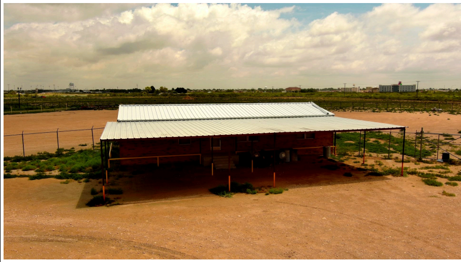
1,568± SF brick field office with covered drive-through canopy.
