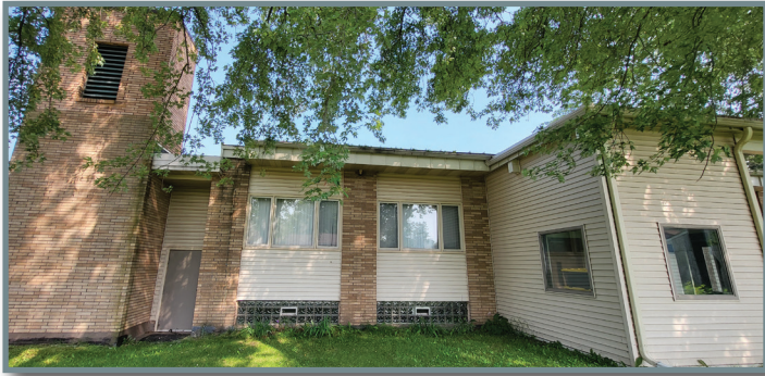
Easy access from the front or rear of the building to the lift for Handicapped Accessibility.
