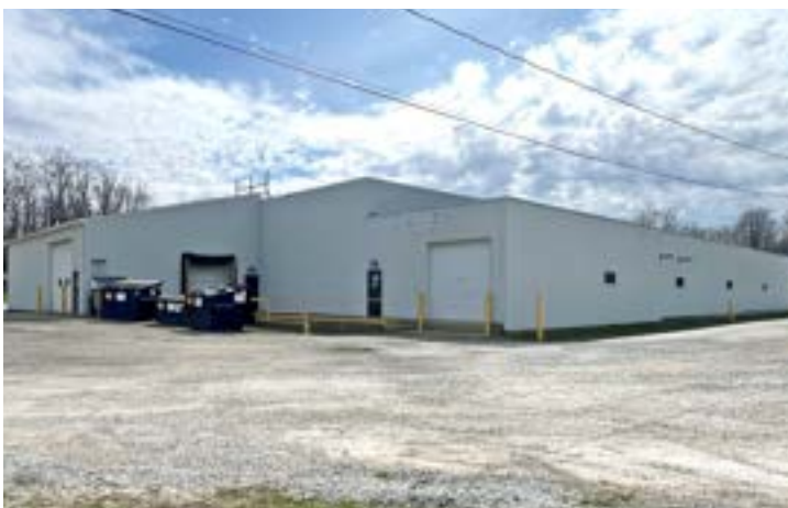
2 Drive-In Overhead Doors (14'W x 12'H & 10'W x 10'H)
