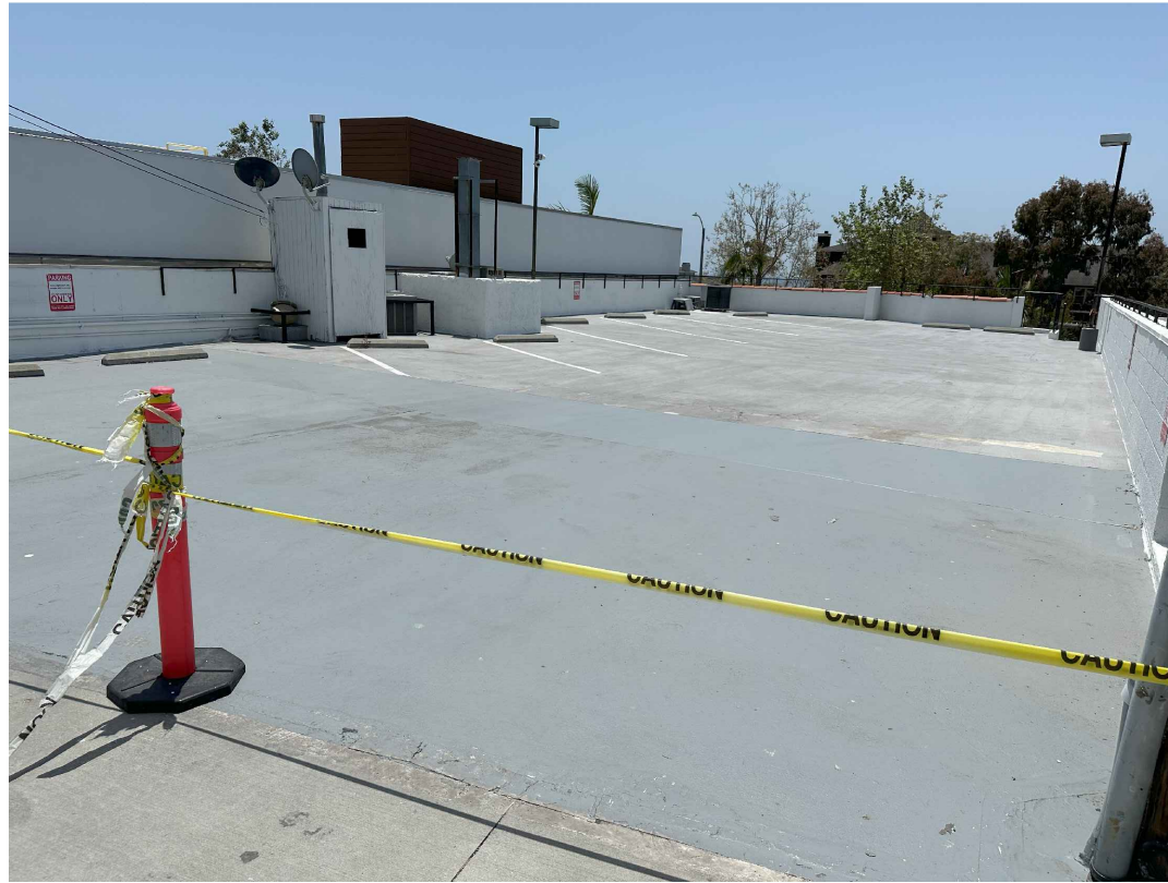
View of Roof from Alley
