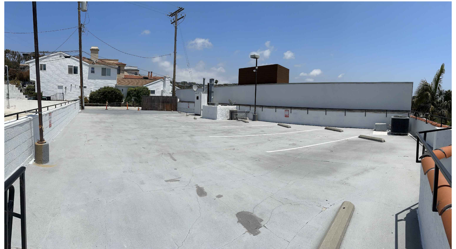
View of Roof from Stairs
