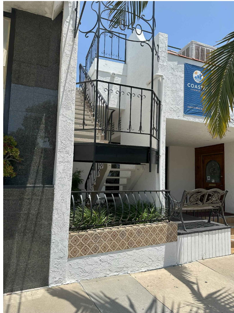
Enlarged View of Existing Stairs
