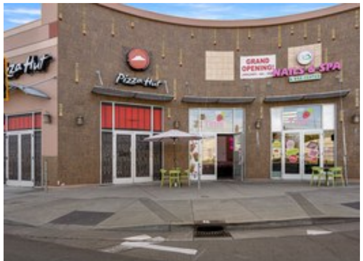
Building Exterior Detail
