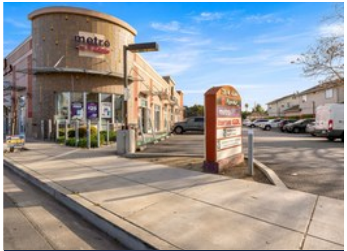
Corner Pylon Sign — All Tenants Listed
