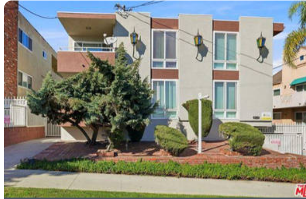
427 East Tamarack Avenue
