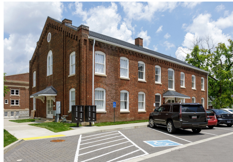
BUILDING D / 6,443 SF
