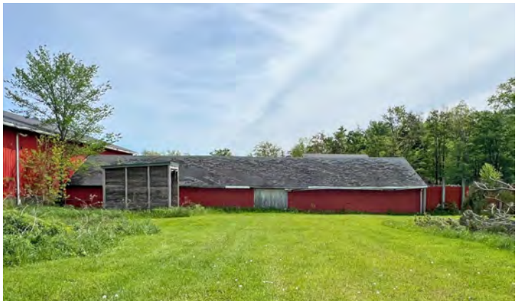
Bldg. 6: 3,672± SF Storage Building
