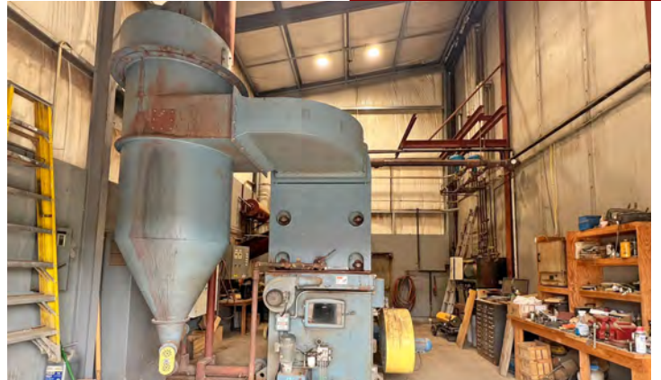
Bldg. 4: 1,749± SF Boiler/Kiln Facility Includes 20' To 25'6" Clear Ceilings
