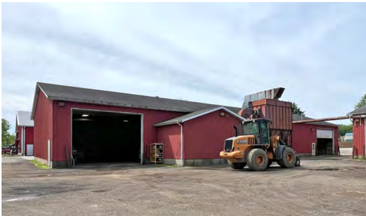
Bldg. 2: 8,824± SF Shop/Warehouse With 16' Clear Ceilings, 2 Overhead Doors: 18'W x 14'H, Reznor Gas Heat & 400 Amp, 480V, 3 Phase Service
