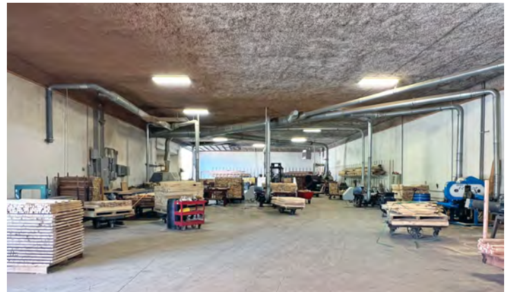
Bldg. 2: 8,824± SF Shop/Warehouse Includes Break Room, Office Area & 3 Restrooms – Built In 1992
