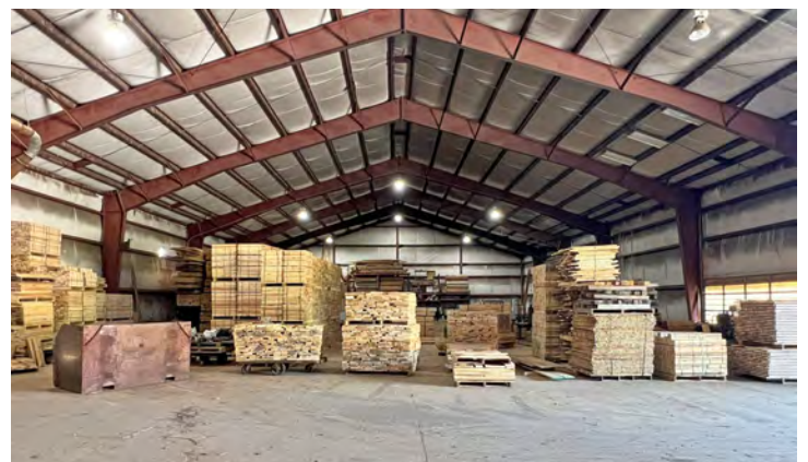
Bldg. 3: 13,200± SF Warehouse Includes 19'8" x 21'3" Storage Room With Mezzanine Storage Above – Built In 1998
