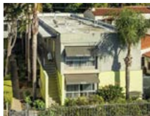
BALBOA FLATS 3533 6th Avenue Hillcrest
