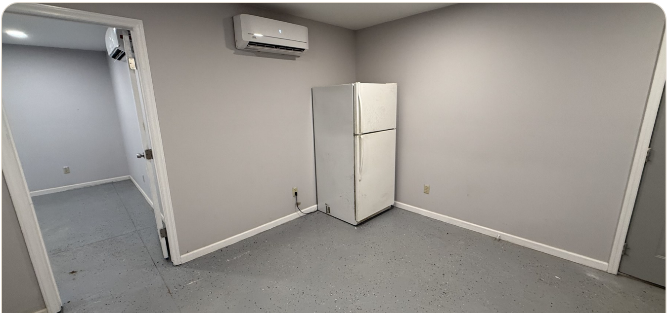
Finished HVAC office/support space
