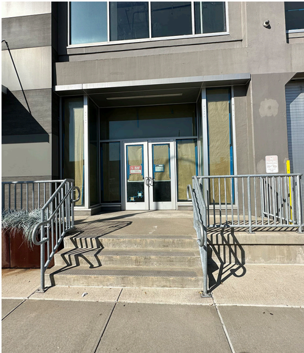
DEDICATED ENTRANCE TO GROUND FLOOR UNIT
