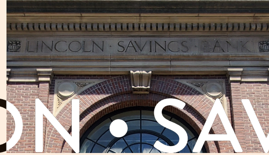
Architectural molding with "Lincoln Savings Bank" engraved
