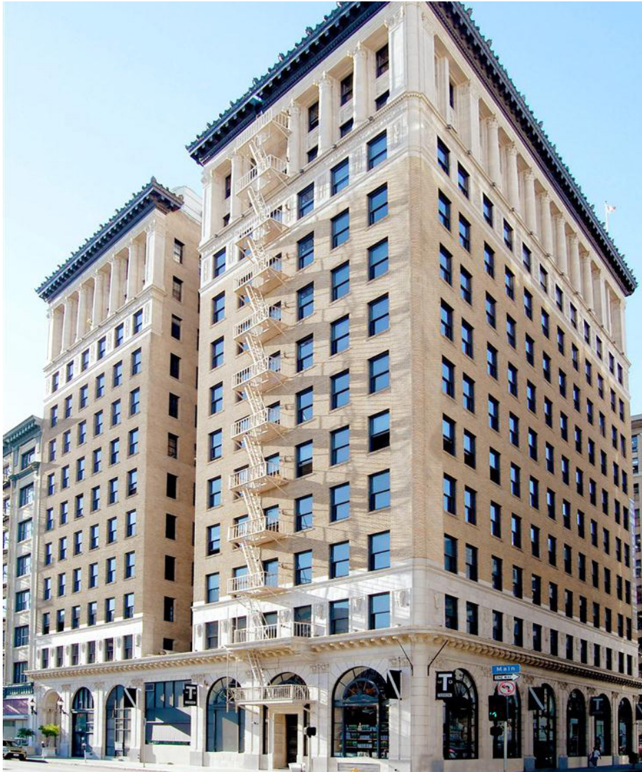
Corner of Main St. & 8th St.
