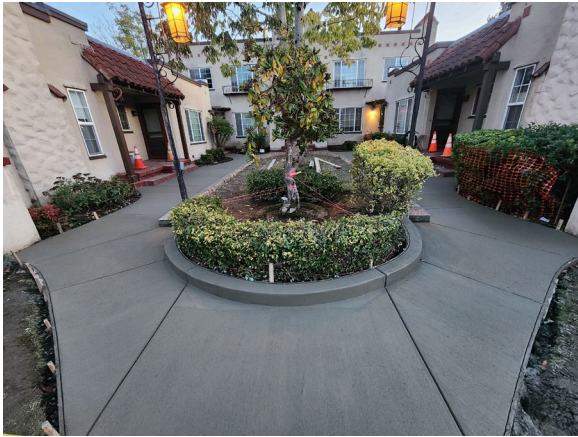
New Concrete Courtyard Walkway 2025
