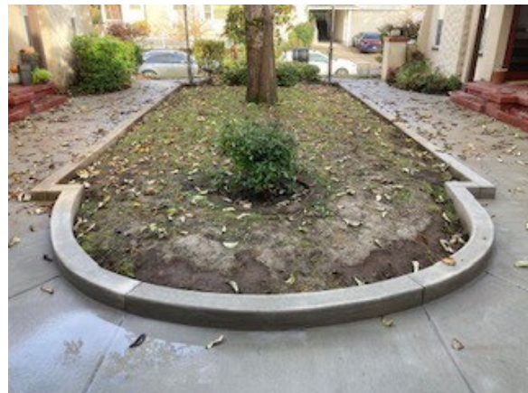
Courtyard Features All New Concrete
