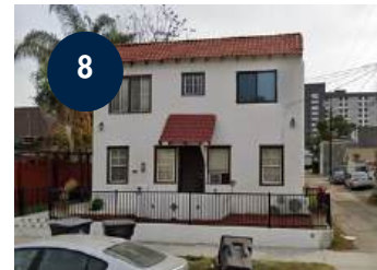
3448 FAIRMOUNT BLVD RIVERSIDE
