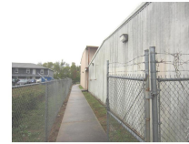
VIEW ALONG REAR OF BUILDING THREE AND FOUR
