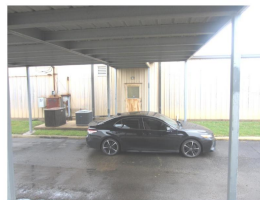
VIEW OF COVERED WALKWAY BETWEEN BUILDING 2 & 1
