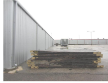
VIEW ALONG WESTERN BOUNDARY LOOKING NORTH
