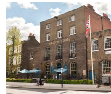
3. Aragon House, (bar, restaurant & boutique hotel)
