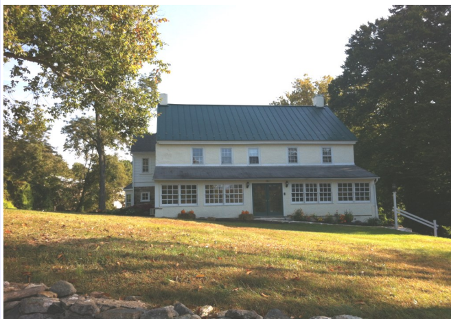
Alternate front view of building.
