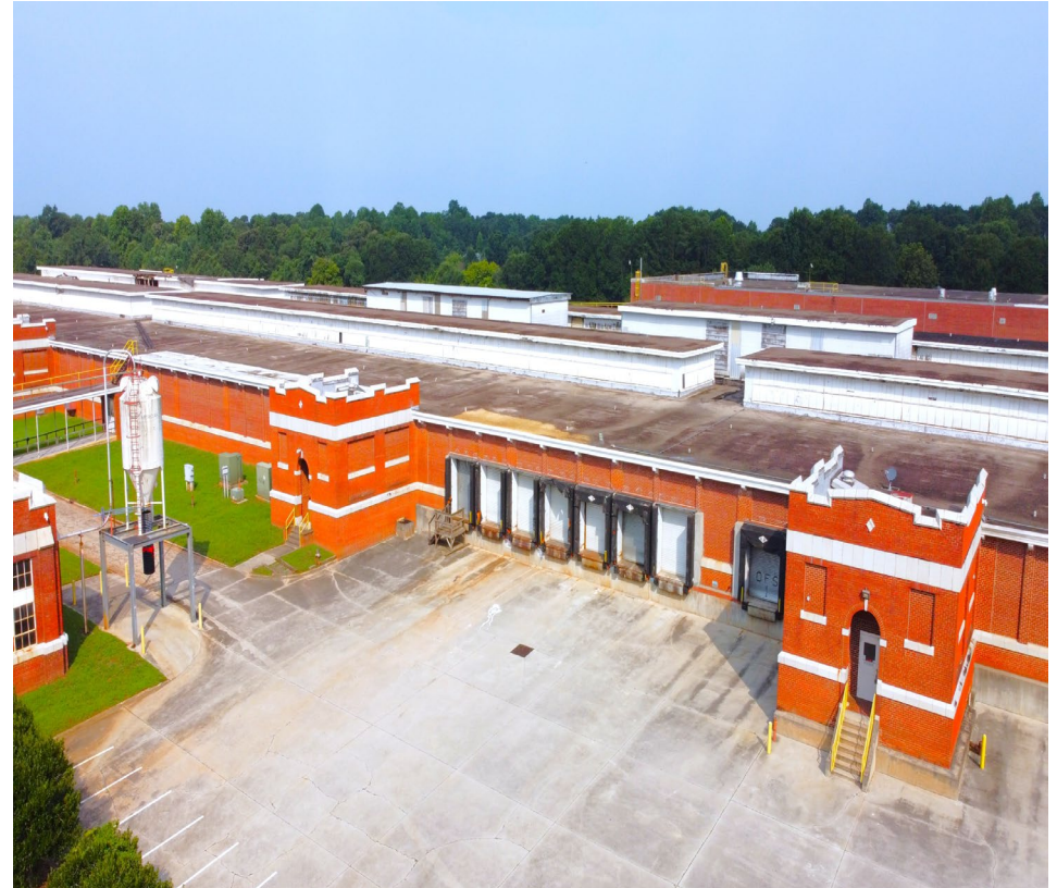
Loading Dock & Warehouse Court
