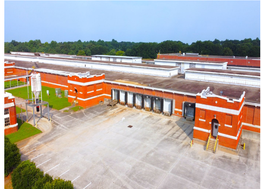
Rear loading court — multiple dock-high doors
