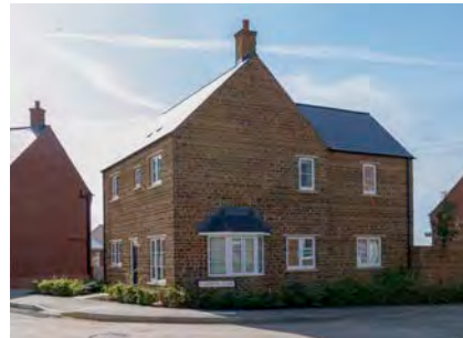
Fig. 1.9 Claydon Close, Hanwell View
