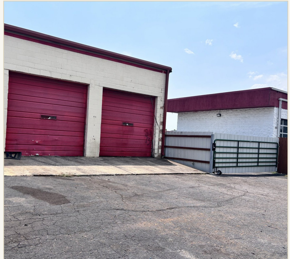
Rear bays — two of the four 12' garage doors
