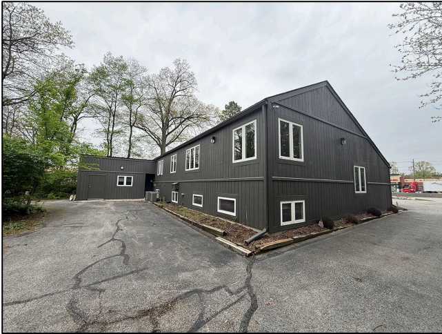
Rear parking lot and access to Office 108
