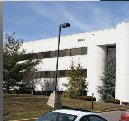
1031 US HIGHWAY 22 BRIDGEWATER, NJ 08807
