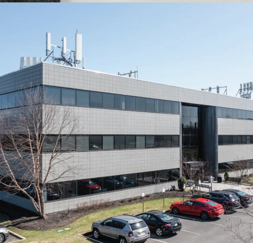
1170 US HIGHWAY 22 BRIDGEWATER, NJ 08807
