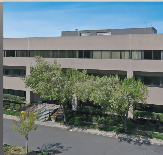
1011 US HIGHWAY 22 BRIDGEWATER, NJ 08807
