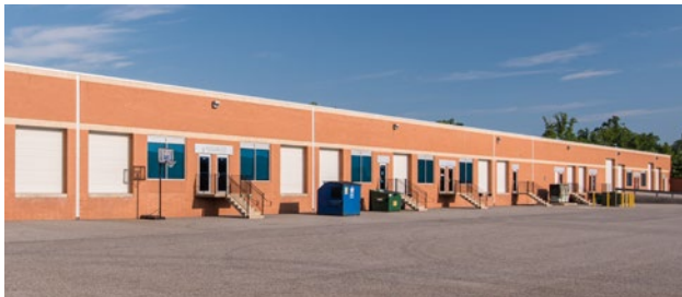
Flex/R&D dock and drive-in loading
