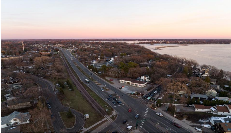
4561 Lake Avenue — aerial view of building, drive lanes, and monument sign
