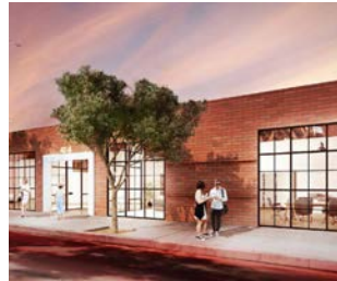
4216 WEST JEFFERSON 11,873 SF creative office
