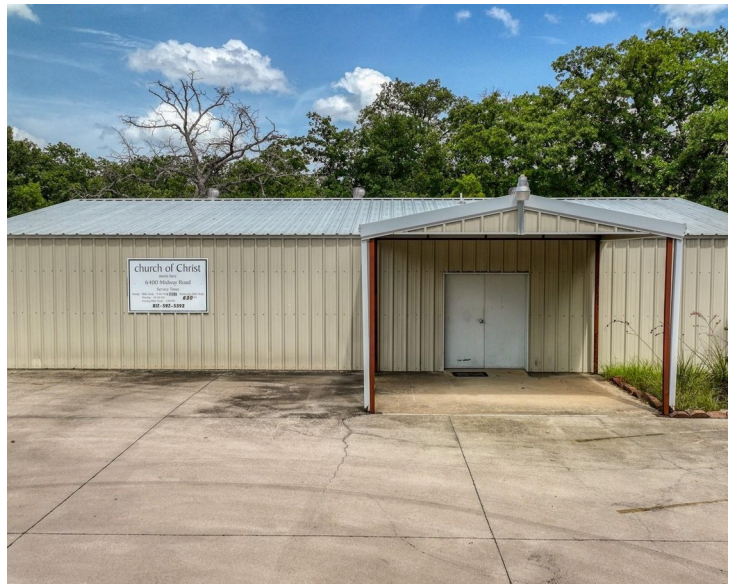
Front elevation — covered entry
