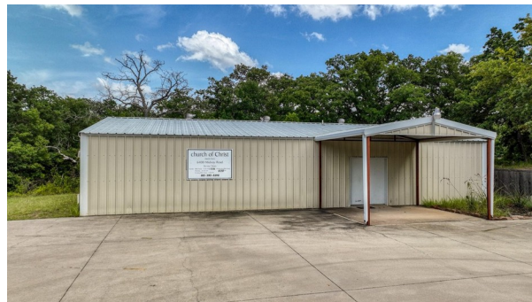
Front elevation and concrete parking apron
