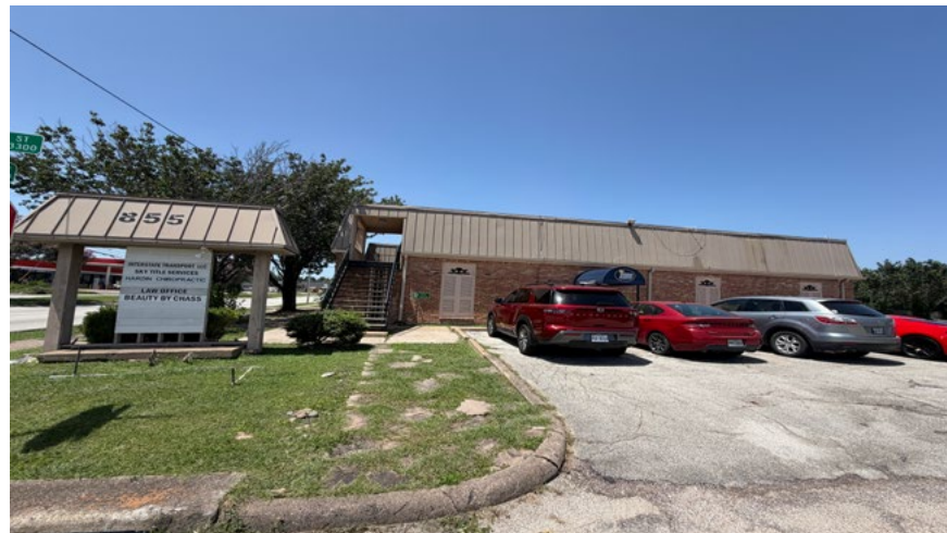
South side of property
