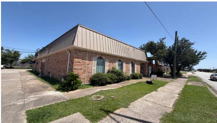
North and west side of property
