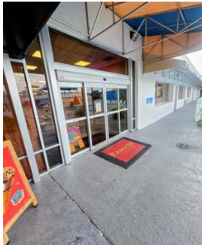
Water Park Entrance to Lobby
