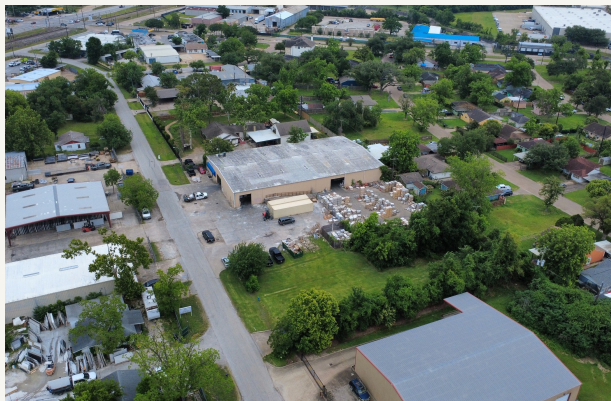
CONCRETE LAYDOWN YARD
