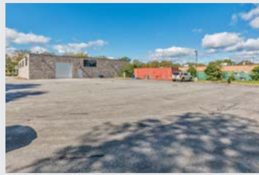
Oversized Yard Space
