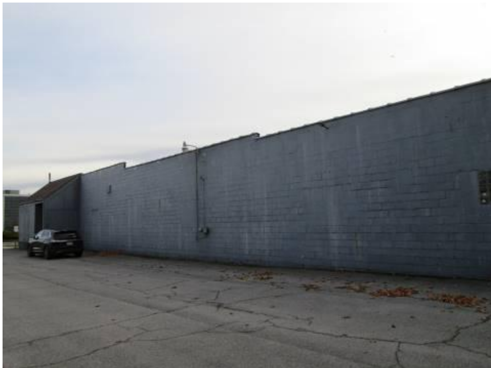
Northeast Side of Building
