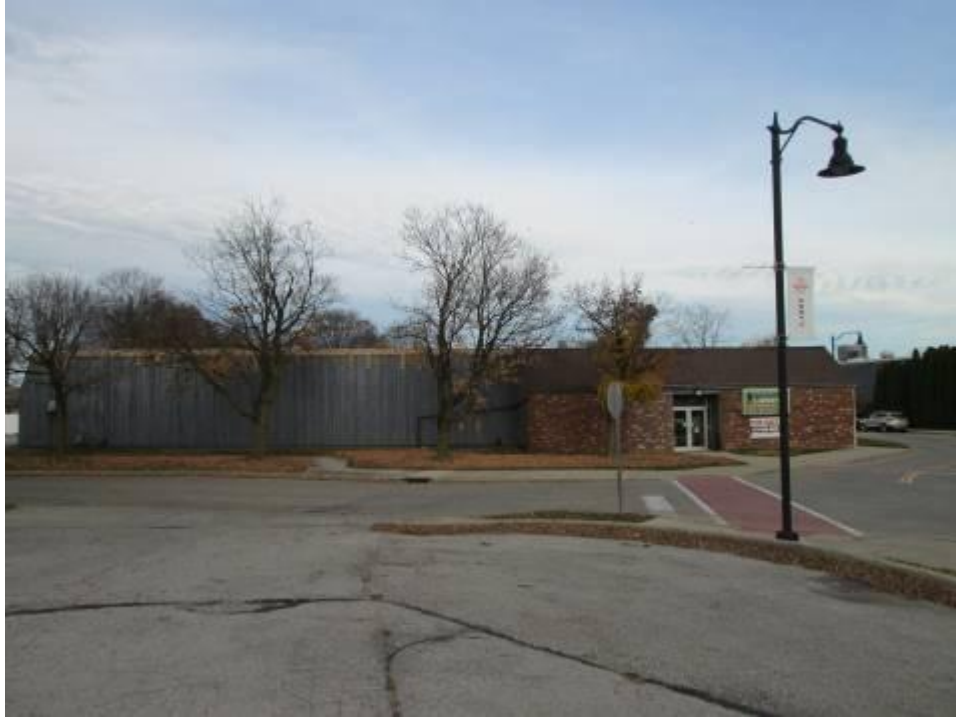
Southwest Side of Building
