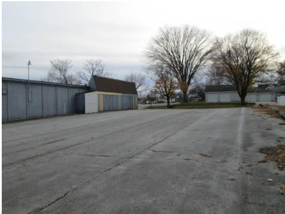
Rear of Building and Rear Parking Lot
