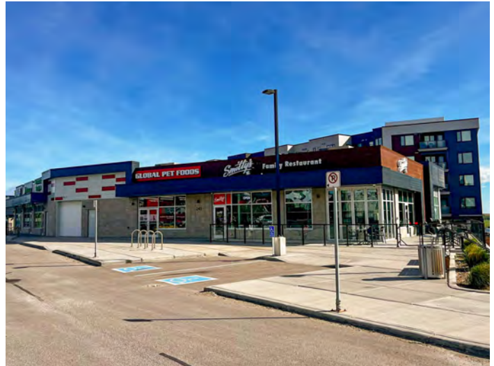
Building K - Upper Level - (Leased)
