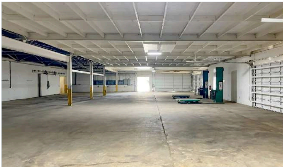
INTERIOR — OPEN WAREHOUSE AND DOCK DOORS
