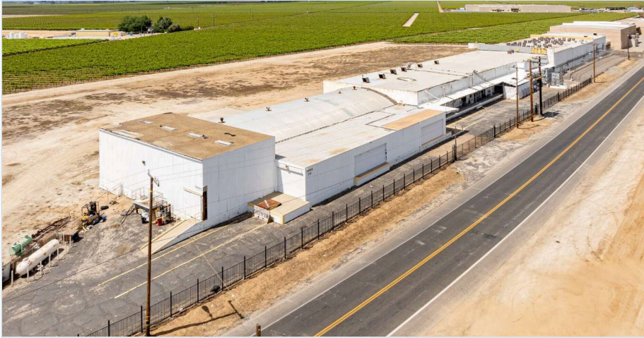
AERIAL — HIGHWAY FRONTAGE AND BUILDING ENVELOPE
