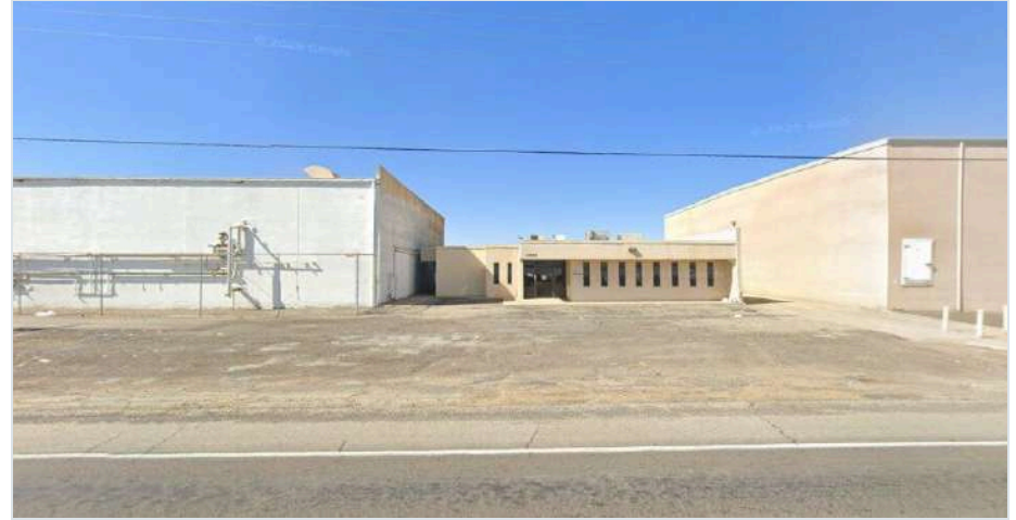
FRONT ELEVATION AND PAVED YARD
