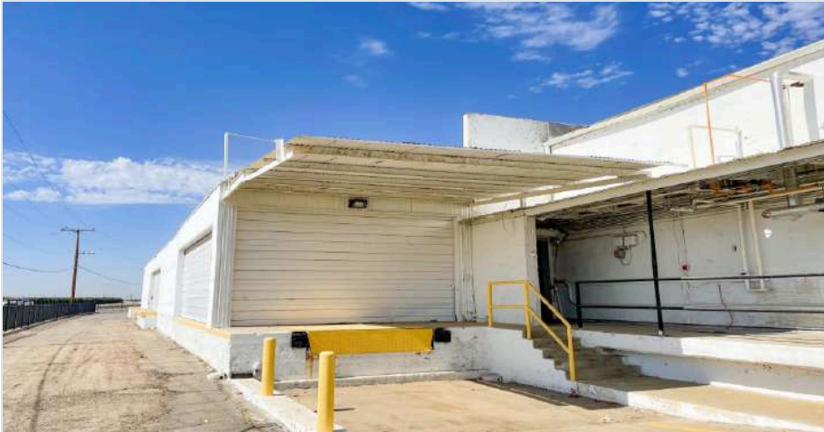
DOCK AND CANOPY LOADING AREA
